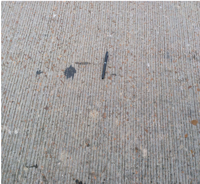
PHOTO 1 Description Typical Deck crack.
