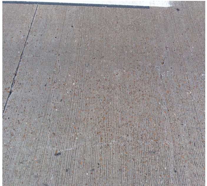
PHOTO 2 Description Typical Deck cracks.
